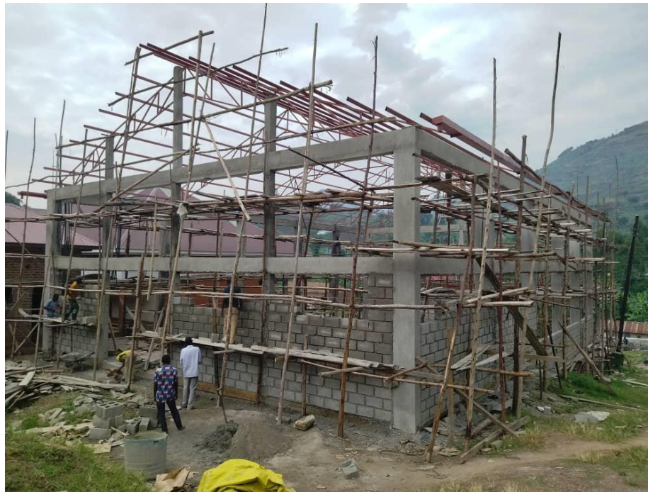
Figure 1: Construction of a modern factory nearing completion
